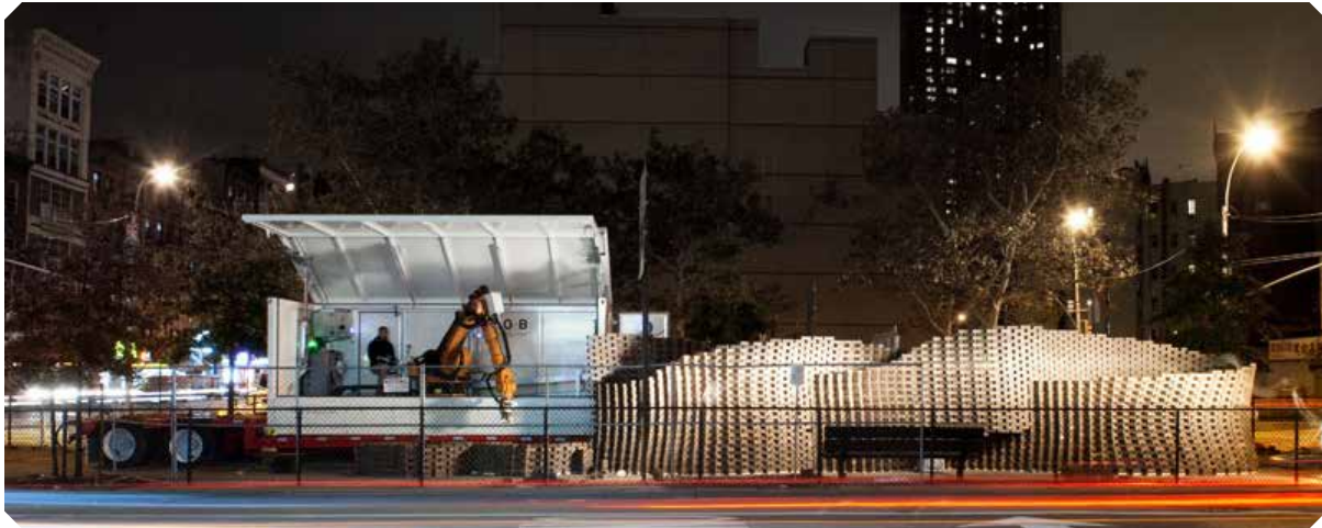
Fig. 1.3. The ROB unit building Pike Loop by Gramazio & Kohler in NYC. (image from Gramazio and Kohler © ETH)
