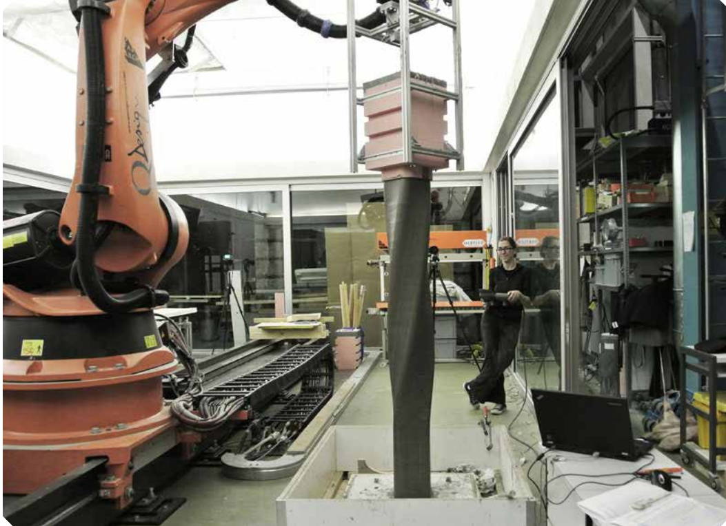
Fig. 1.15. Dynamic Concrete Casting by Gramazio & Kohler has very real construction potentials (Gramazio & Kohler © ETH).
